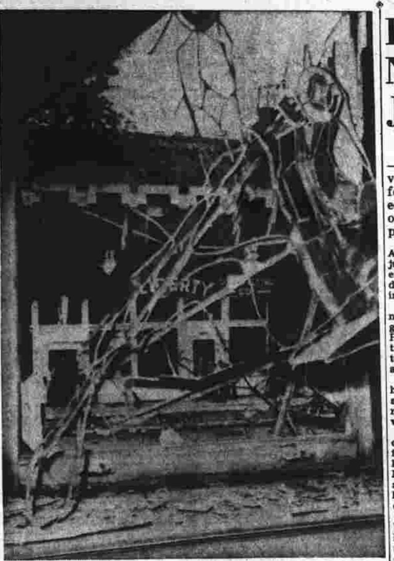
Bomb blast in Birmingham, Ala., 6th Avenue Baptist church broke and twisted this stained glass window. (AP Photofax.)
